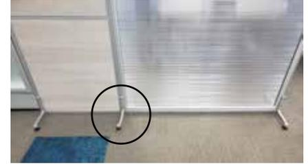
**\*When using hinges on connecting panels a wheel can be added to one of the panels in place of the foot so the panel moves more freely. (see below).**
